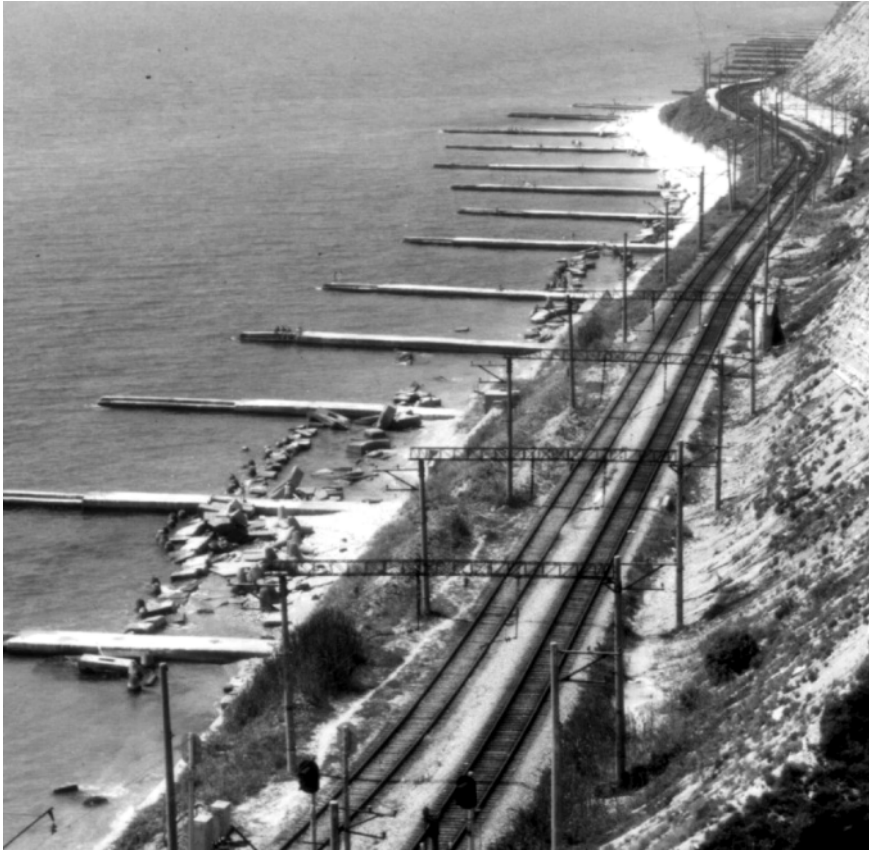
Fig.2.Empty sections between bunas in the area of Tuapse – Sochi railroad.
