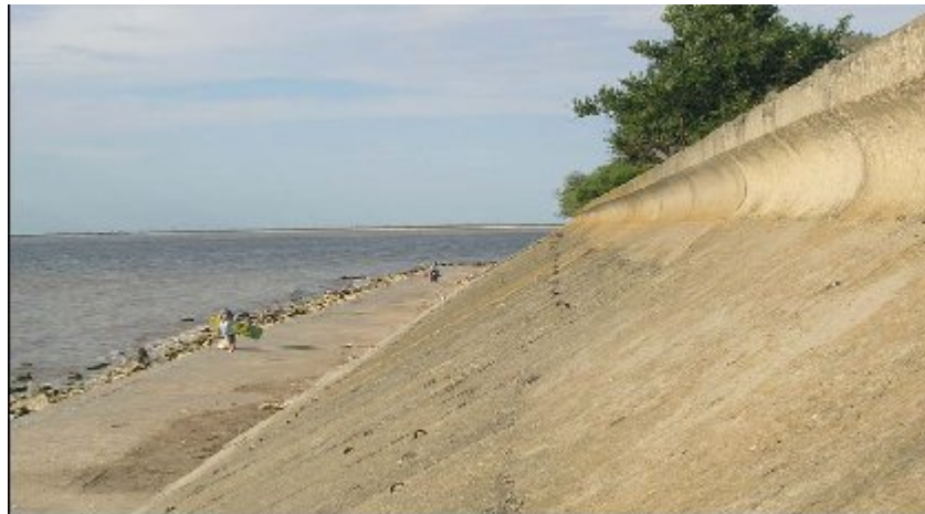
Figure 8: Coast protection near bowery Morozovsky
