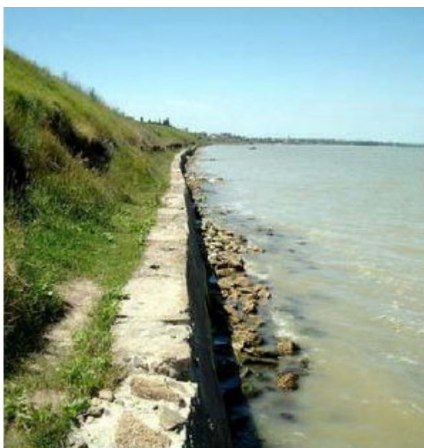
Figure 15: Coast protection complex of the railway roadbed
