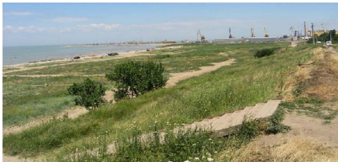
Figure 14: Coast protection complex, s. Eysk
