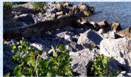
каменная наброска 1982 – 1985 the stone revetment constructed in 1982 - 1985
